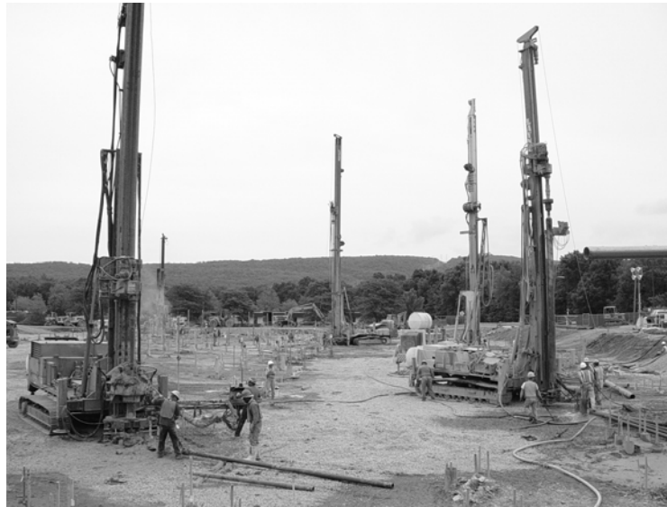
Figure 1. Intense micropile construction site, with multiple rigs working 24 hours per day
